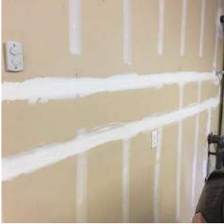
Walls & Windows (4/6) 02/02/2021 2:06 PM
