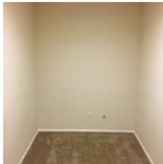
Walls & Windows (3/3) 02/02/2021 1:54 PM
