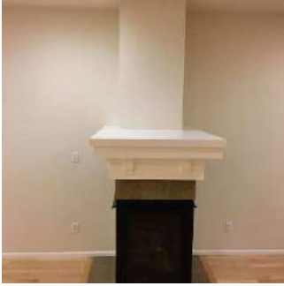
Walls & Windows (3/5) 02/02/2021 1:25 PM
