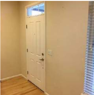
Walls & Windows (1/4) 02/02/2021 1:19 PM
