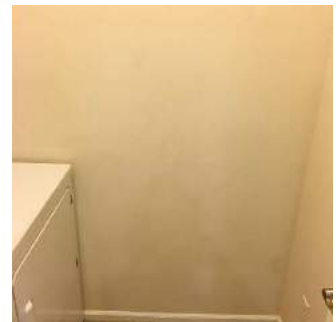
Walls & Windows (4/4) 02/02/2021 1:42 PM
