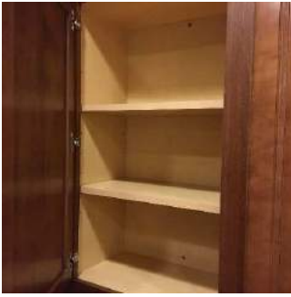
Kitchen cabinets / Closet / etc (2) (3/16) 02/02/2021 1:32 PM
