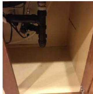
Sink & Underneath Sink (1/2)
