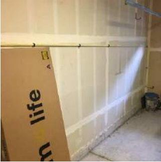
Walls & Windows (5/6) 02/02/2021 2:06 PM
