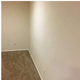
Walls & Windows (2/3) 02/02/2021 1:54 PM
