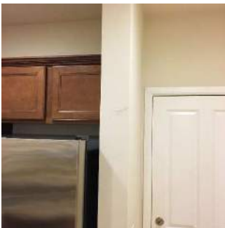
Walls & Windows (1/2) 02/02/2021 1:29 PM
