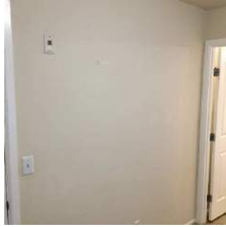
Walls & Windows (1/4) 02/02/2021 1:44 PM
