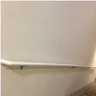
Walls & Windows (1/3) 02/02/2021 1:22 PM
