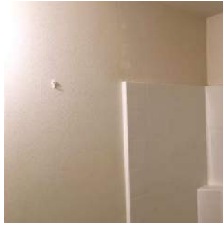
Walls & Windows (4/7) 02/02/2021 1:50 PM
